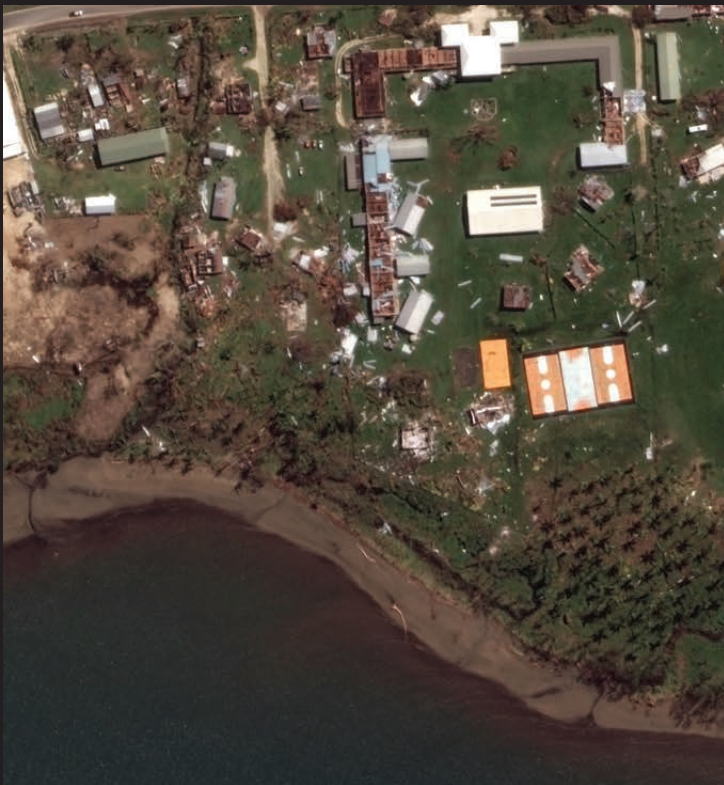
Maxar satellite imagery of damage from Cyclone Harold in Vanuatu, taken 10 April 2020 with WorldView-2. Satellite imagery ©2021 Maxar Technologies.
